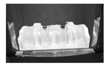
b) Place the left hand front pebble rail moulding onto the front ceramic rail support and locating pins as shown below in Fig. 11
